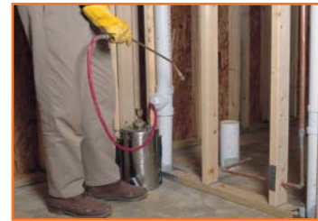
Treating interior bathroom walls.
