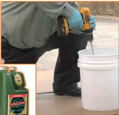
Use a drill and impeller to mix Bora-Care with Mold-Care
