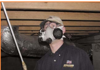
Treating a subfloor controls mold and prevents dry rot and insect infestation that also accompany moisture problems.
