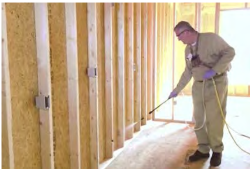
Bora-Care is applied to your homes by your pest company during the dried-in phase of construction.
