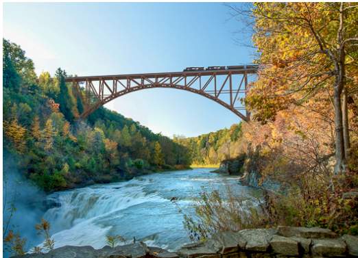
Photo Courtesy of Modjeski & Masters, Inc.
