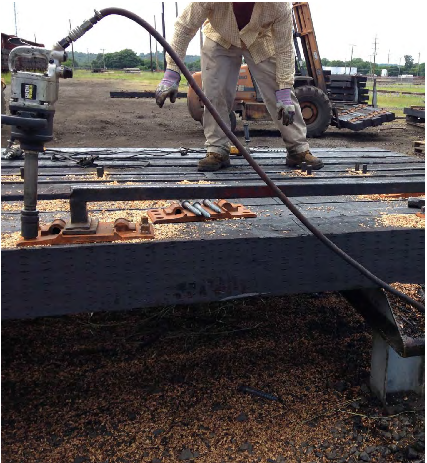
FIGURE 10. Drilling holes in a treated tie can expose untreated wood. Whenever possible, holes, daps, etc., should be cut before pressure treatment. If drilling or fabricating must be done after treatment, preservative must be applied locally at that time. Such “field” treatments are required under AWP Standard M4, and copper naphthenate at 2 percent Cu is standardized for ground contact applications.
