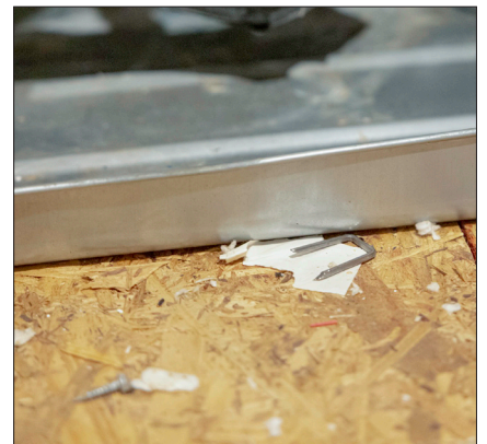
Debris such as screws, staples, and nails can end up hidden in insulation and damage vacuum or harm applicators during removal. Ensure that precautions are taken.
