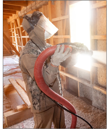
A PMP applying insulation with appropriate PPE.
