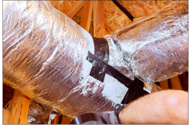
Damaged ductwork should be patched and sealed prior to installation.
