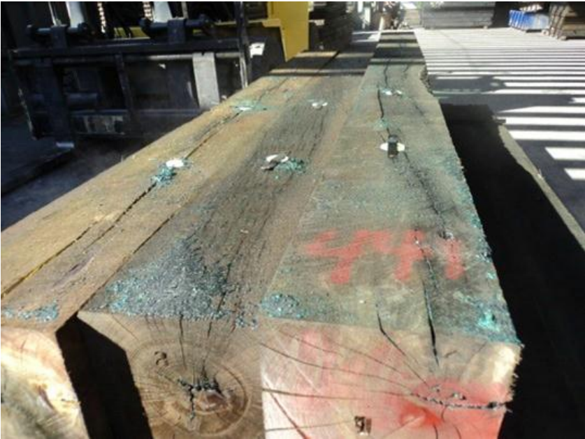
Figure 4. Bridge ties after Bouton treatment.
