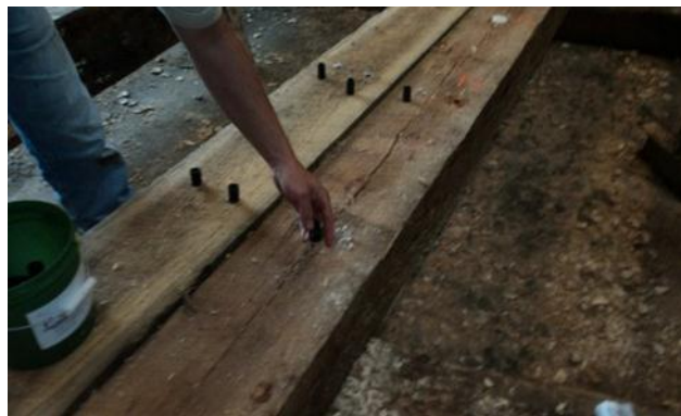
Figure 1. Insertion of 7/8" (2.2cm) sleeves in the 13/16" (2.1cm) holes
