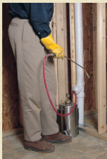
Bora-Care is applied to all structural wood to help prevent drywood infestations.
