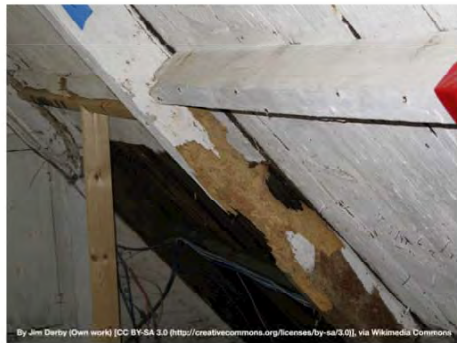
Powderpost beetle damage to the sapwood of a pitch pine rafter on Cape Cod, Massachusetts
