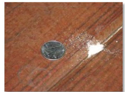
Porch damage from powderpost beetles with dime for size
