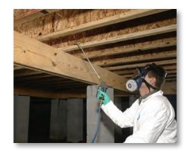
In homes with crawl spaces, the entire subfloor can be treated to help prevent termites, wood boring beetles and wood decay fungi.
