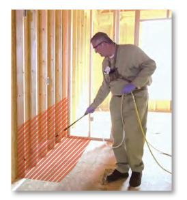
The 2-foot band treatment is needed to protect the structure from termites. This gives termite and general pest protection at the base of walls where pests tend to build nests if they get access to a home. Bora-Care also protects against entry over treated concrete and around plumbing penetrations.
