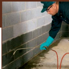
Treat the foundation walls in a crawl space or basement.
