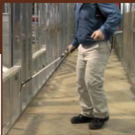
Treat the interior stud walls.
