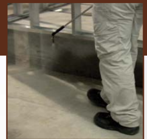
Treat abutting slabs and expansion joints.
