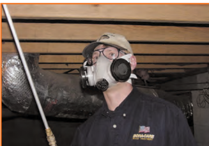
Treating a subfloor controls mold and prevents dry rot and insect infestation that also accompany moisture problems.
