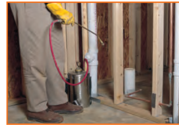
Treating interior bathroom walls.
