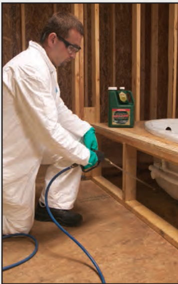
Applying Bora-Care with Mold-Care to a water-damaged home will kill existing mold and prevent mold from reoccurring. Remember, nothing can stop mold from growing if the conducive conditions are not corrected.
