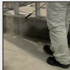
Treat abutting slabs and expansion joints.
