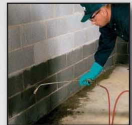
Treat the foundation walls in a crawl space or basement.
