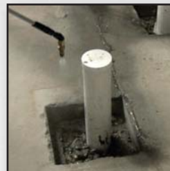
Treat the concrete and plumbing penetrations on slab structures.
