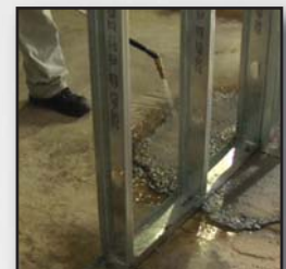
Treat the studs, concrete, and cracks.
